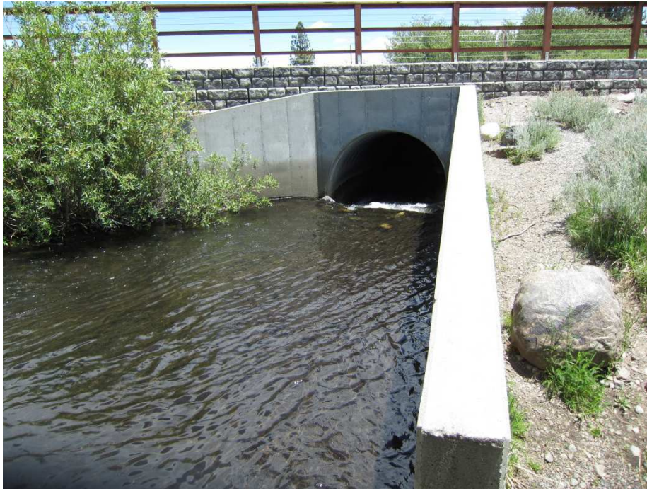
Photo 6: Culvert where Mammoth Creek flows under Minaret Rd.
