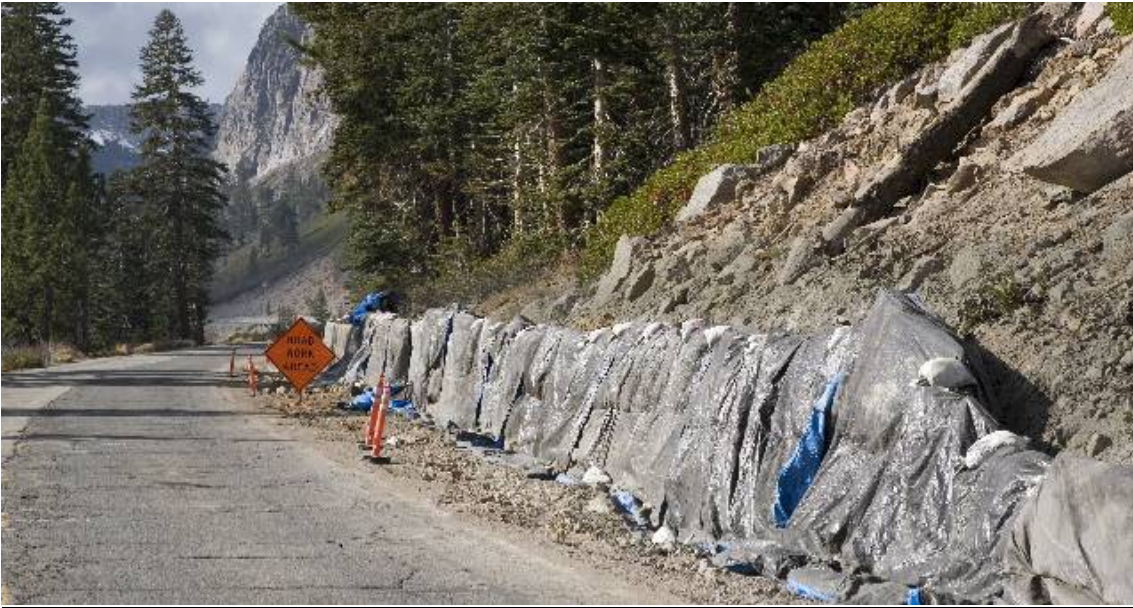
Figure 4-3. Lake Mary Path (under construction)
