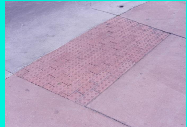
Figure 4.1 Curb Ramp located at Meridian Blvd. and Old Mammoth Road
