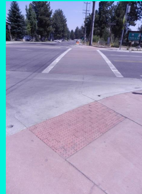
Figure 5.9 This intersection demonstrates a positive example of intersection geometry showing an intersection which is symmetrical with the proper striping and curb ramps.
