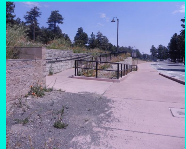
Figure 4.2 ADA Accessible Ramp located on the south side of Main Street near Lupin Street
