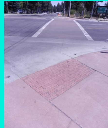
Figure 5.14 Crosswalks and curb ramps
