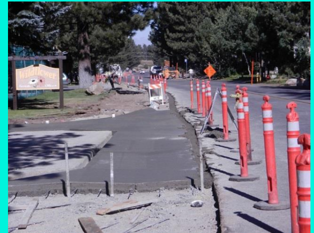
Figure 5.11 Construction zone located on Sierra Nevada Road. The construction area uses minimal amount of space and allows for traffic to pass including pedestrians and bicyclists.
