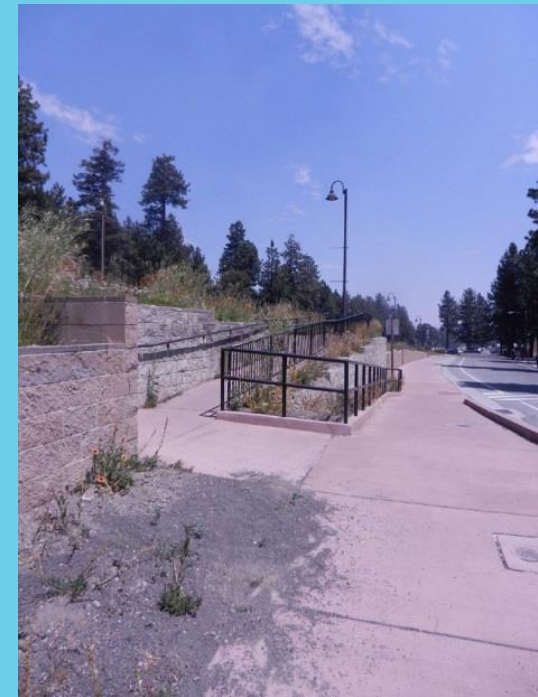
Figure 4.3 ADA-compliant Ramp located on the south side of Main Street
