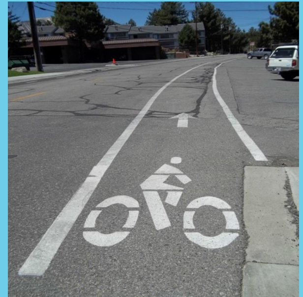
Figure 5.4 There are a number of arterial and collector roads that need Class II bicycle facilities or repainting.
