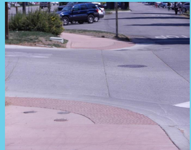
Figure 4.4 ADA-compliant Curb Ramps
