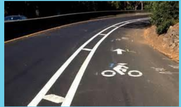
Figure 5.5 A buffered bicycle lane provides additional separation from vehicle traffic. In weather conditions where it is difficult to see, such as sun or fog, a textured bicycle lane alerts drivers if they are crossing out of their lane.
