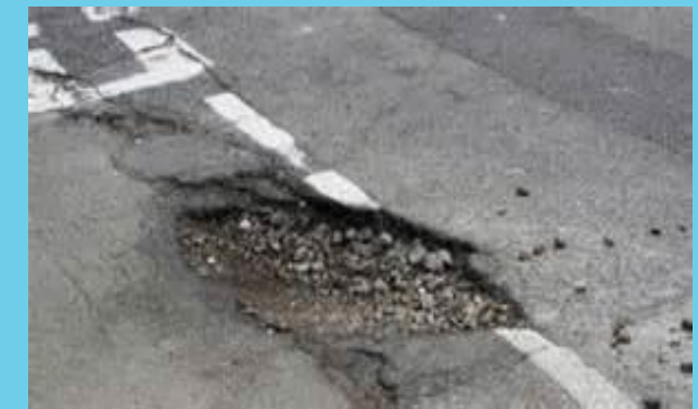
Figure 3.34 Potholes
