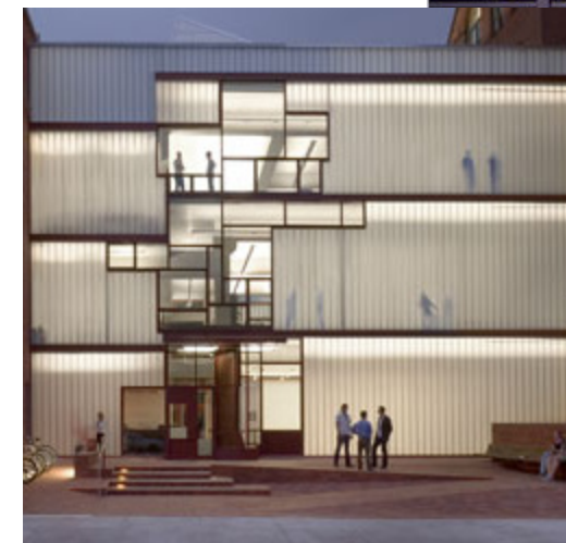
Examples of Channel Wall
