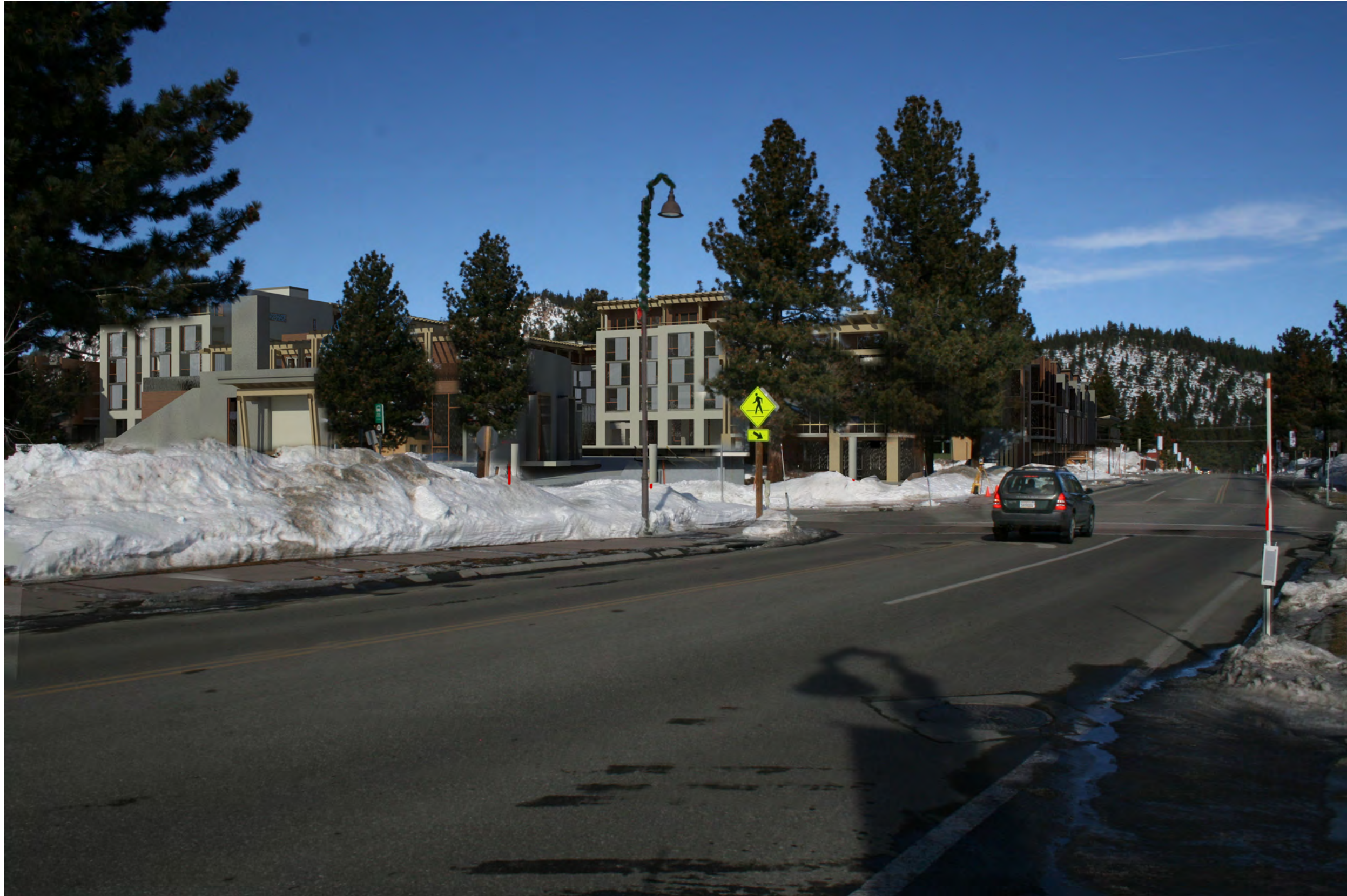
View of SE Corner Looking North on Old Mammoth Road
