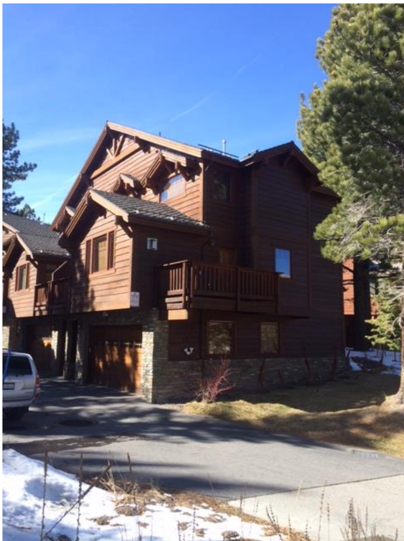
Grayfox Project, 59 Hillside Drive: Mountainside Colors and Materials
