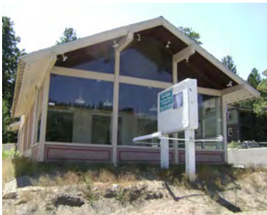
Low lease rates for commercial retail space, due in part by the recession, results in lower projected project values.
