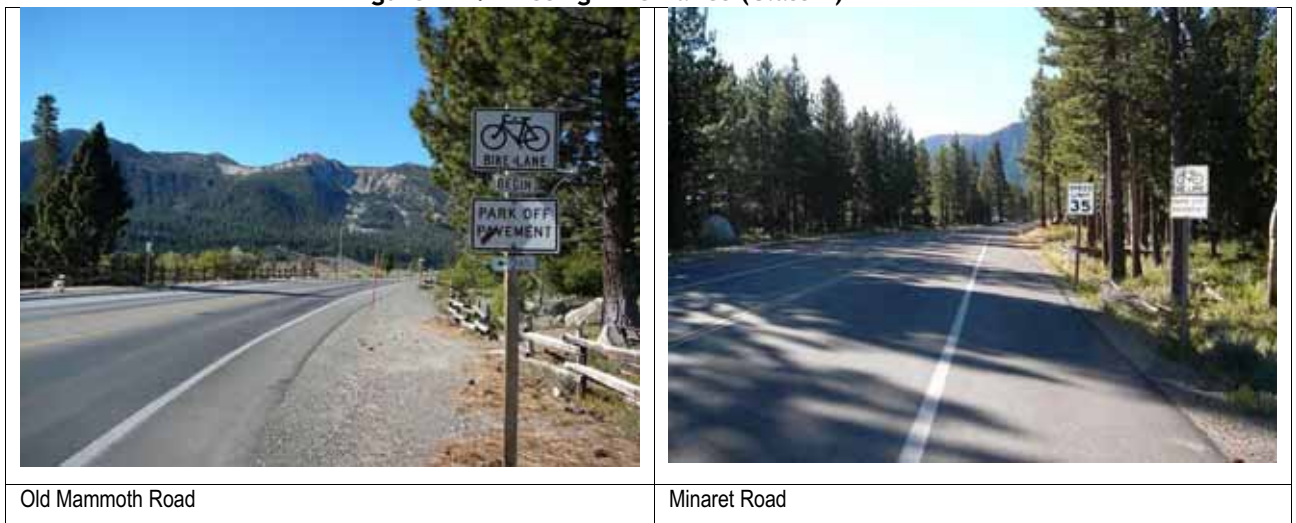
Figure 2-4. Existing Bike Lanes (Class II)
