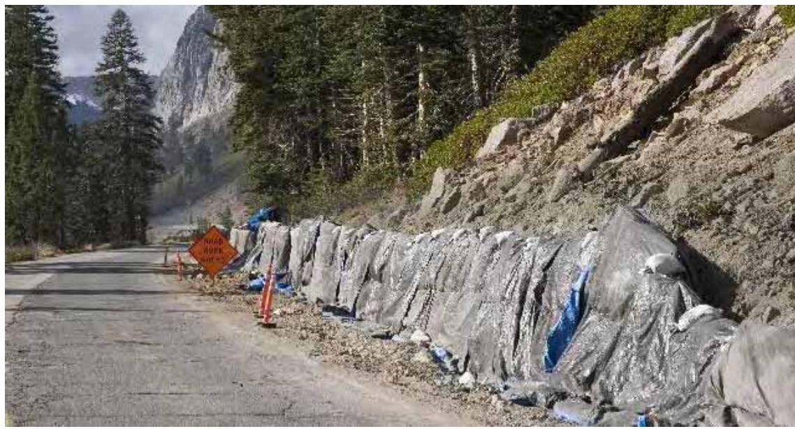
Figure 4-3. Lake Mary Path under construction
