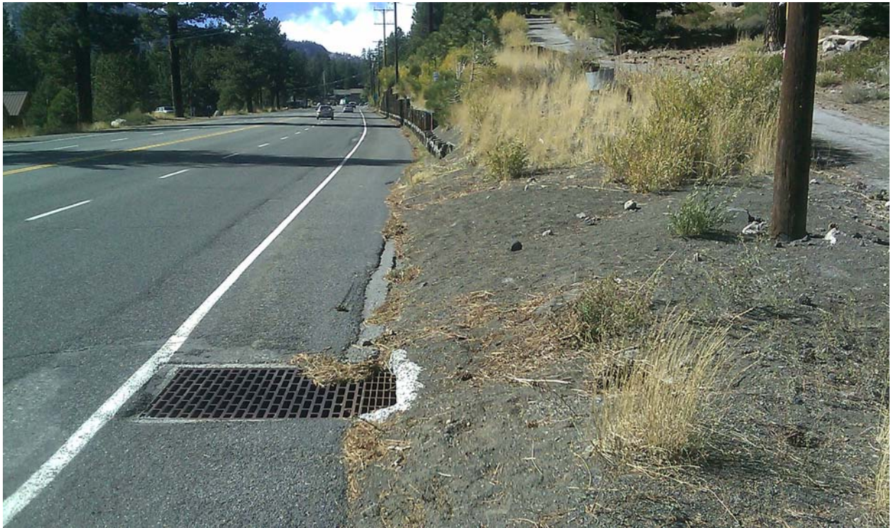
Photo 57. View looking at stormdrain inlet located on Main Street (State Route 203) at Mountain Boulevard.
