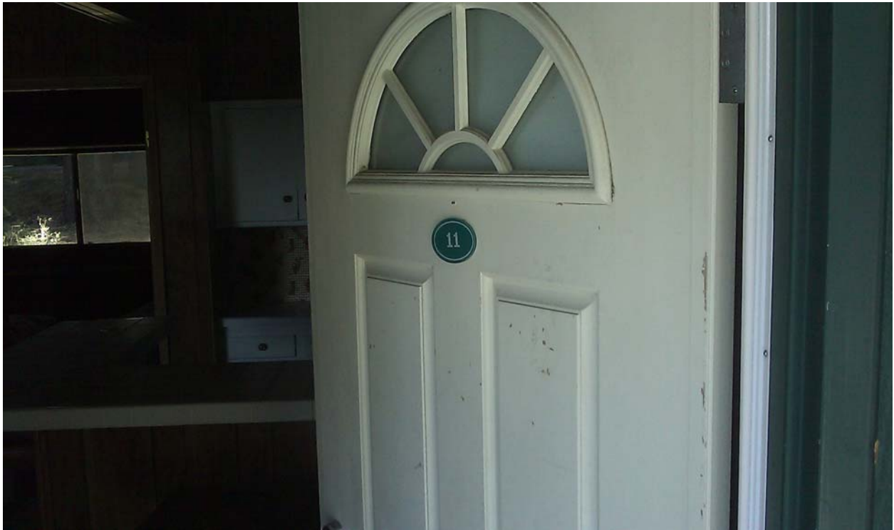
Photo 9. View looking west at entry to Unit 11 of the Royal Pines Resort (west building).
