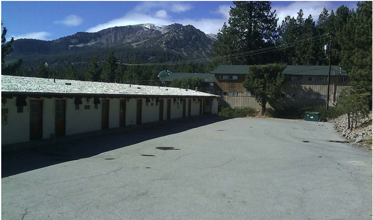
Photo 27. View looking southwest at north (back) side of Swiss Chalet; note 3-phase electrical transformers on power pole (far right).
