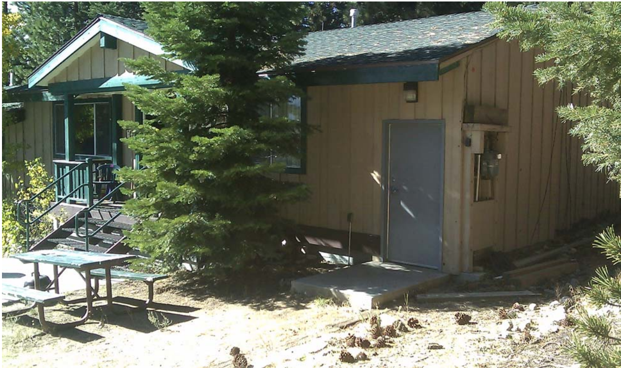
Photo 5. View looking southwest at Royal Pines Resort (west building) maintenance room entry.
