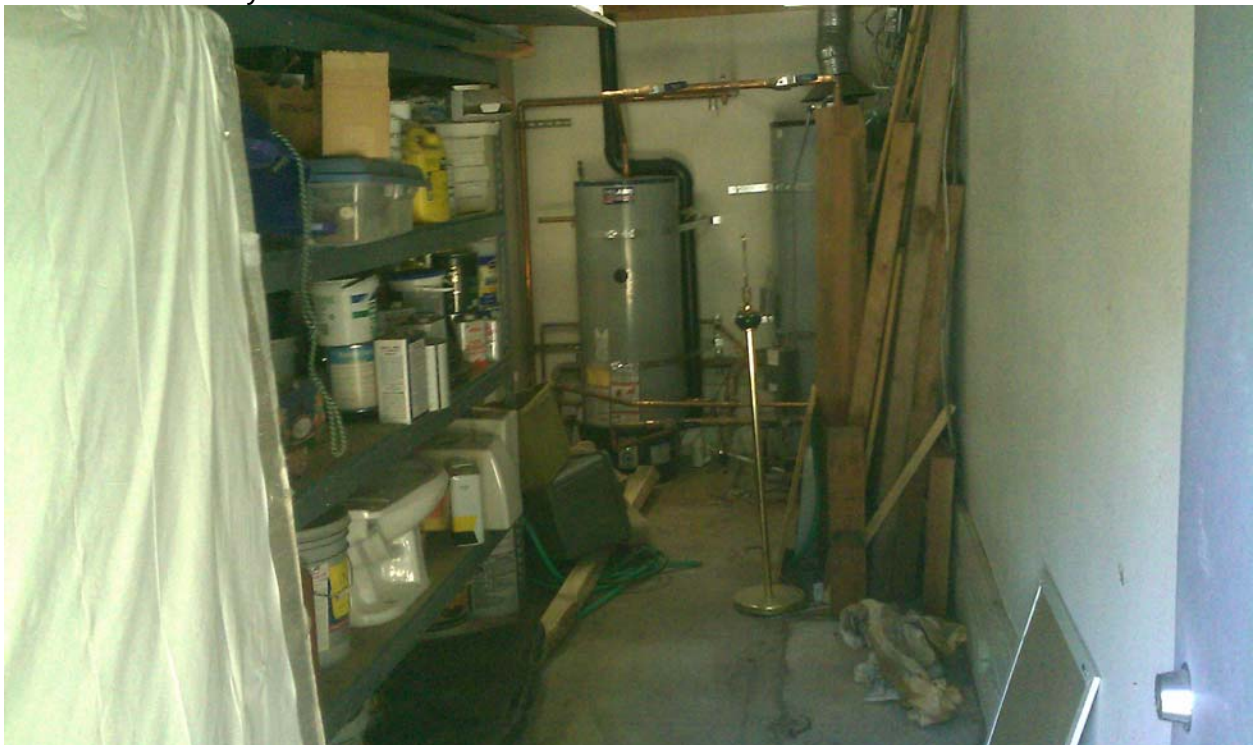
Photo 6. View looking west inside maintenance room.
