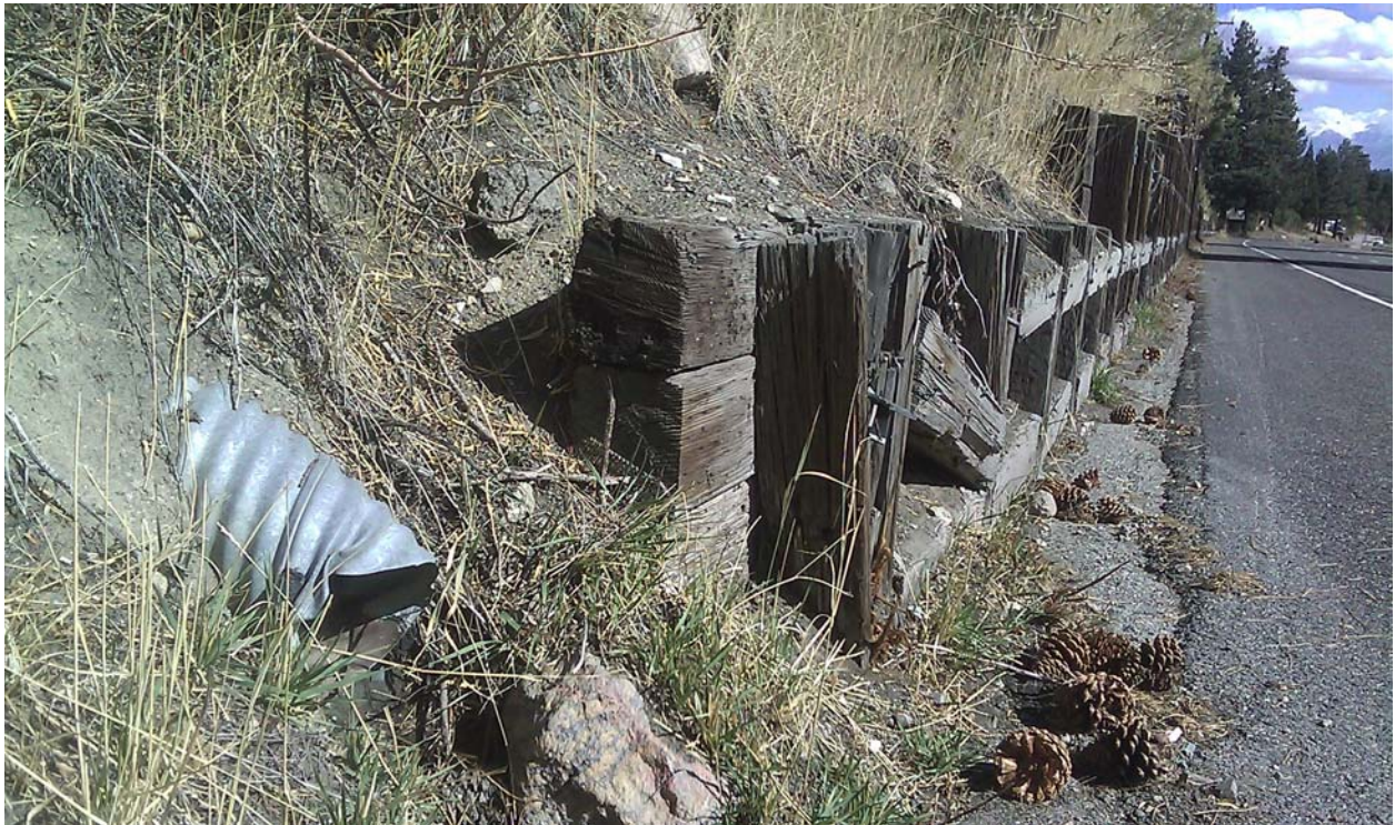
Photo 58. Close-up view of corrugated metal pipe (CMP) stormdrain outlet onto Main Street from Swiss Chalet.
