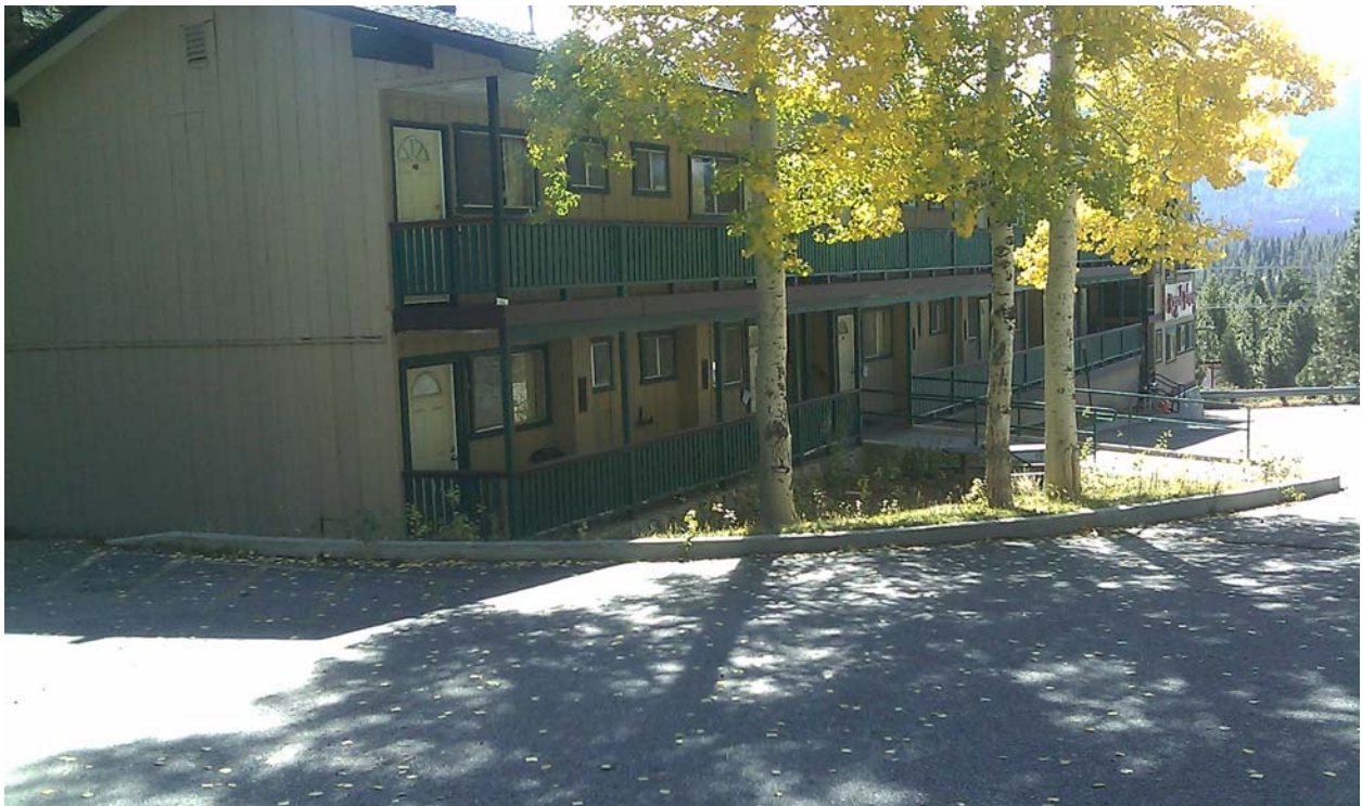
Photo 14. View looking southeast at Royal Pines Resort (east building) from parking lot.
