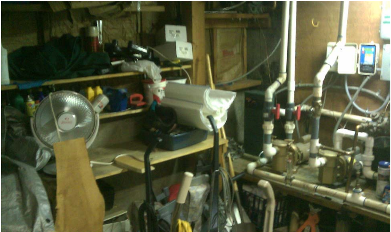
Photo 35. Northeast view inside maintenance room.
