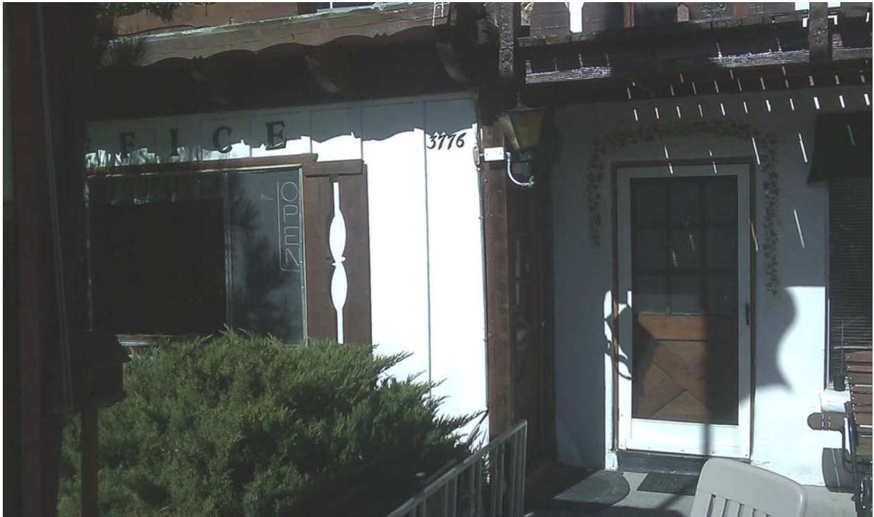
Photo 29. View looking north at office entry to Swiss Chalet from View Point Road/parking area.
