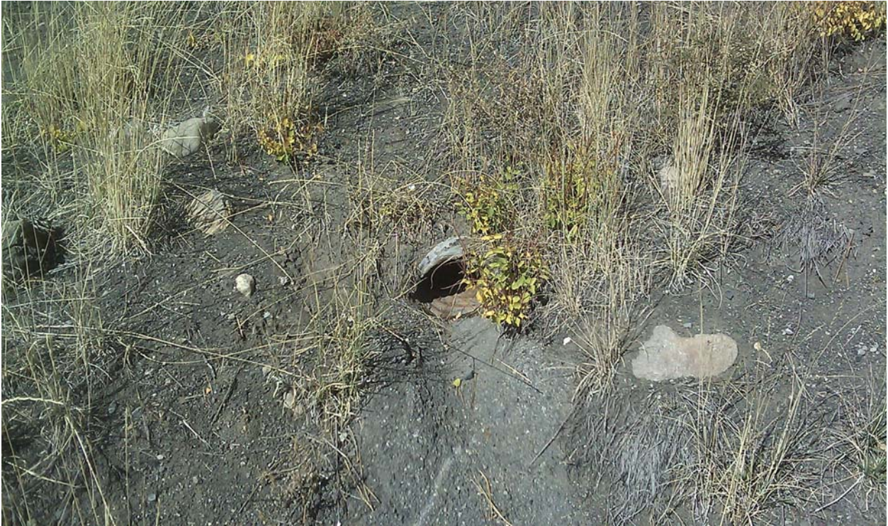
Photo 59. Close-up view of CMP stormdrain outlet onto Main Street from Royal Pines Resort.
