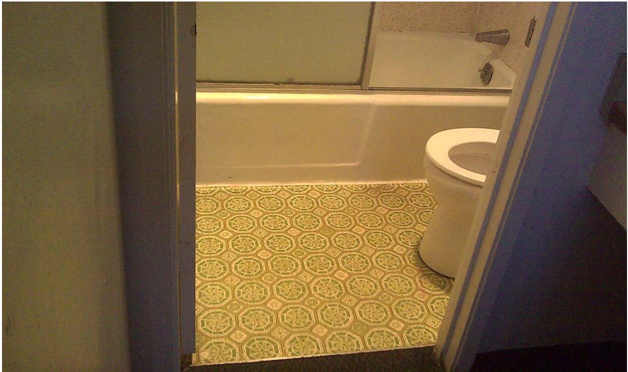
Photo 23. View of bathroom floor tiling inside Unit 18 composed of PACM.
