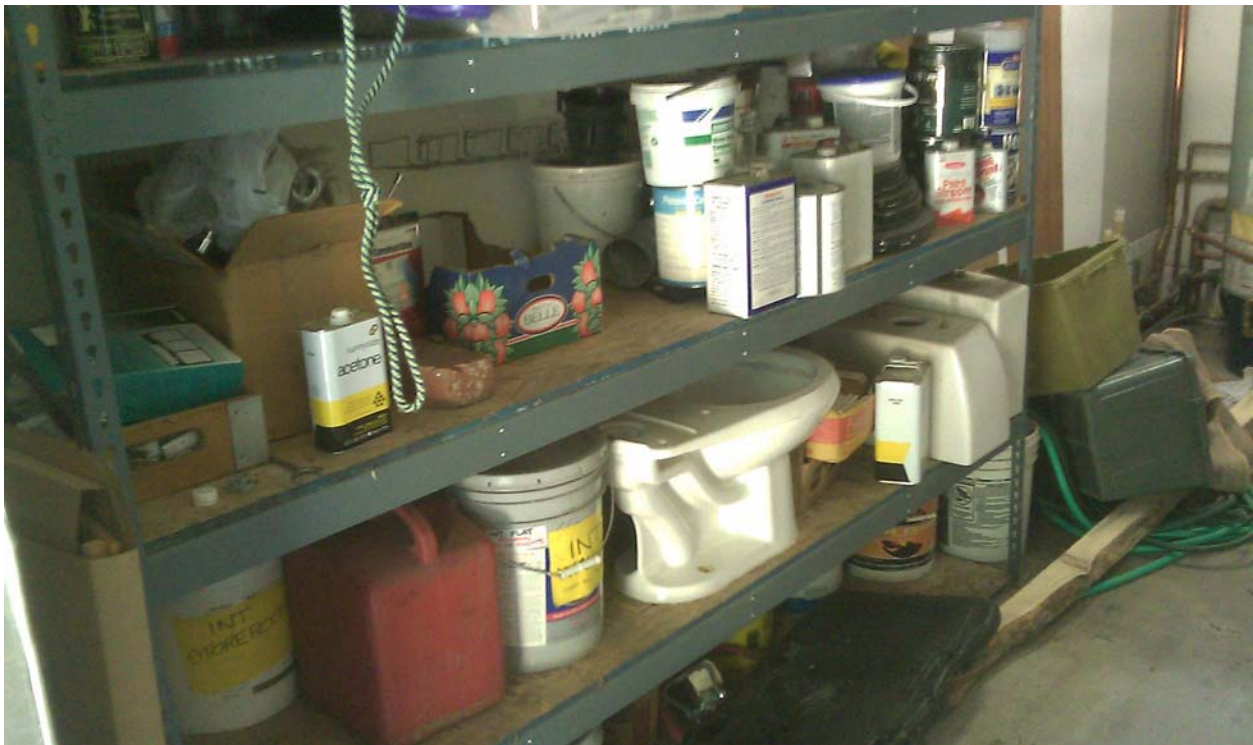
Photo 8. Storage shelves on south wall of maintenance room.
