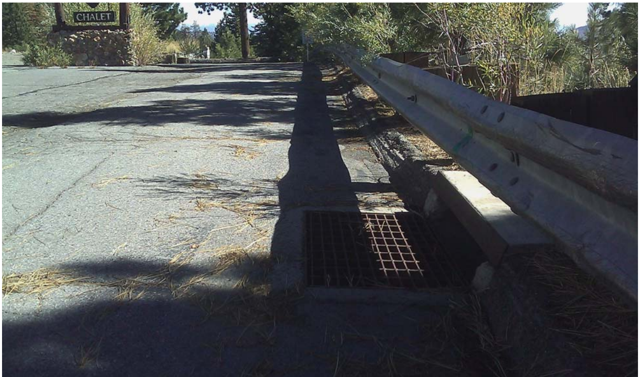
Photo 56. View looking close-up at eastern stormdrain inlet located on View Point Road south of Swiss Chalet.
