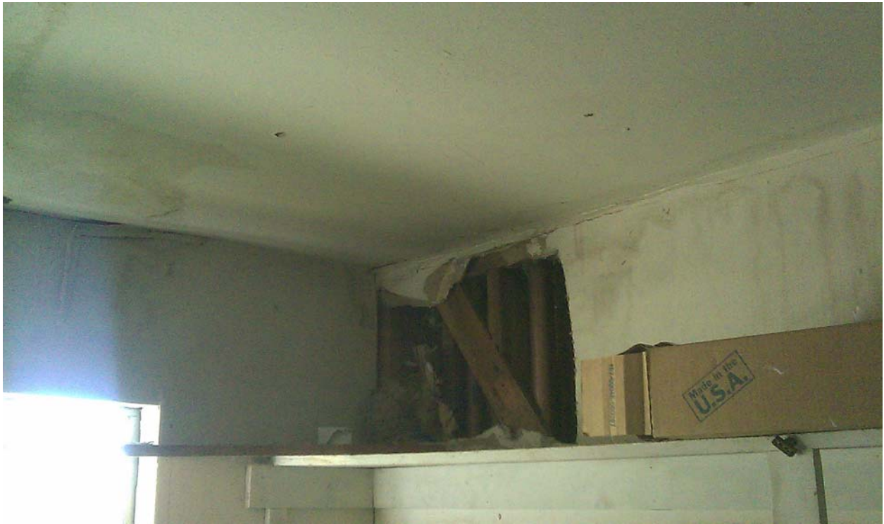
Photo 17. View of "sheet rock" ceiling and walls inside east building maintenance room composed of PACM.
