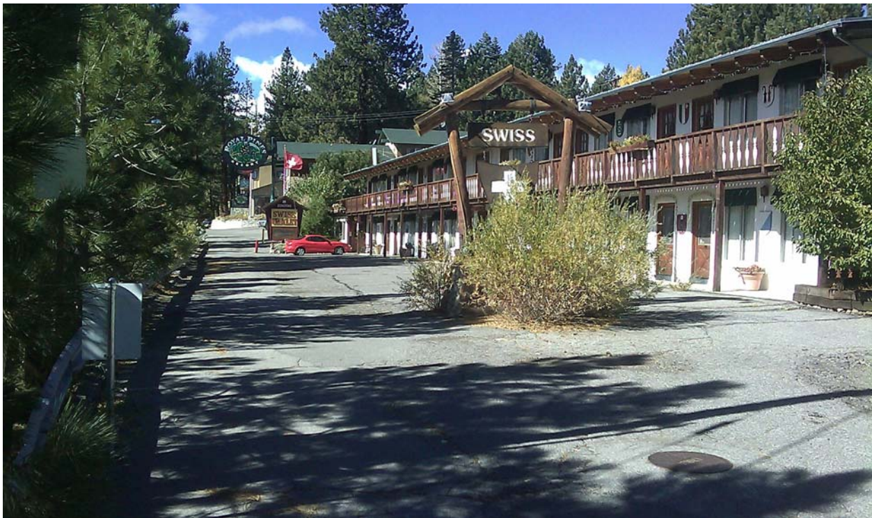
Photo 26. View looking west at Swiss Chalet from View Point Road.
