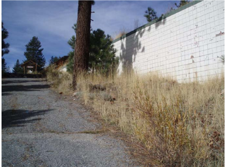
Retaining walls within the Mammoth View Project Area were used to create level construction pads and roads for previous development. 11-5-2010
