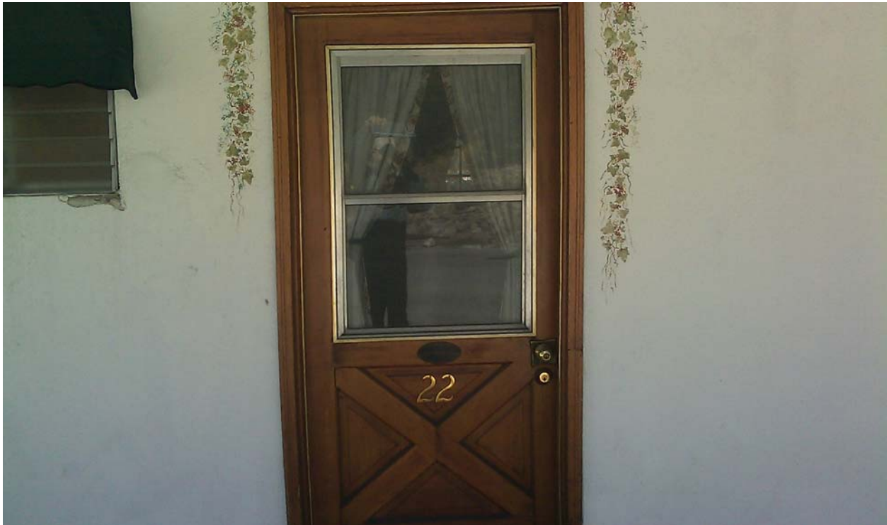
Photo 43. View looking north at entry to Unit 22 of Swiss Chalet from parking area.
