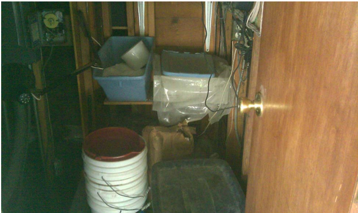
Photo 50. View inside maintenance/storage room.
