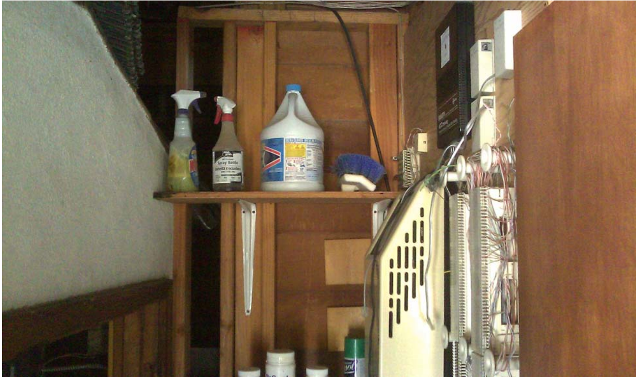
Photo 49. View inside maintenance/storage room.
