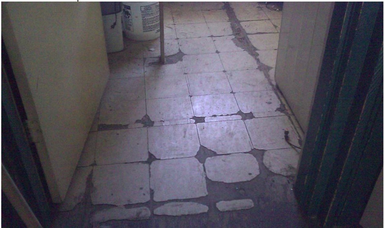
Photo 18. View of floor tiling inside east building maintenance room composed of PACM.
