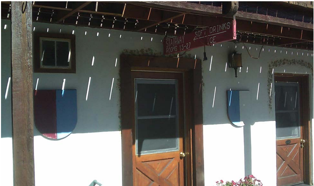
Photo 36. View looking northeast at laundry room access to Swiss Chalet from View Point Road/parking area.
