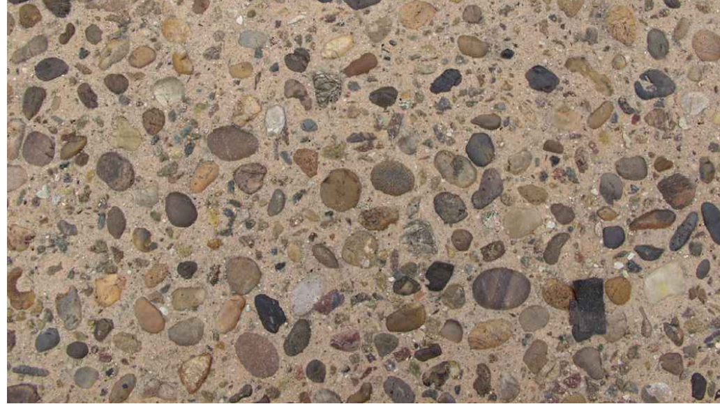
16.SEEDED CONCRETE AT NATURAL PATH
