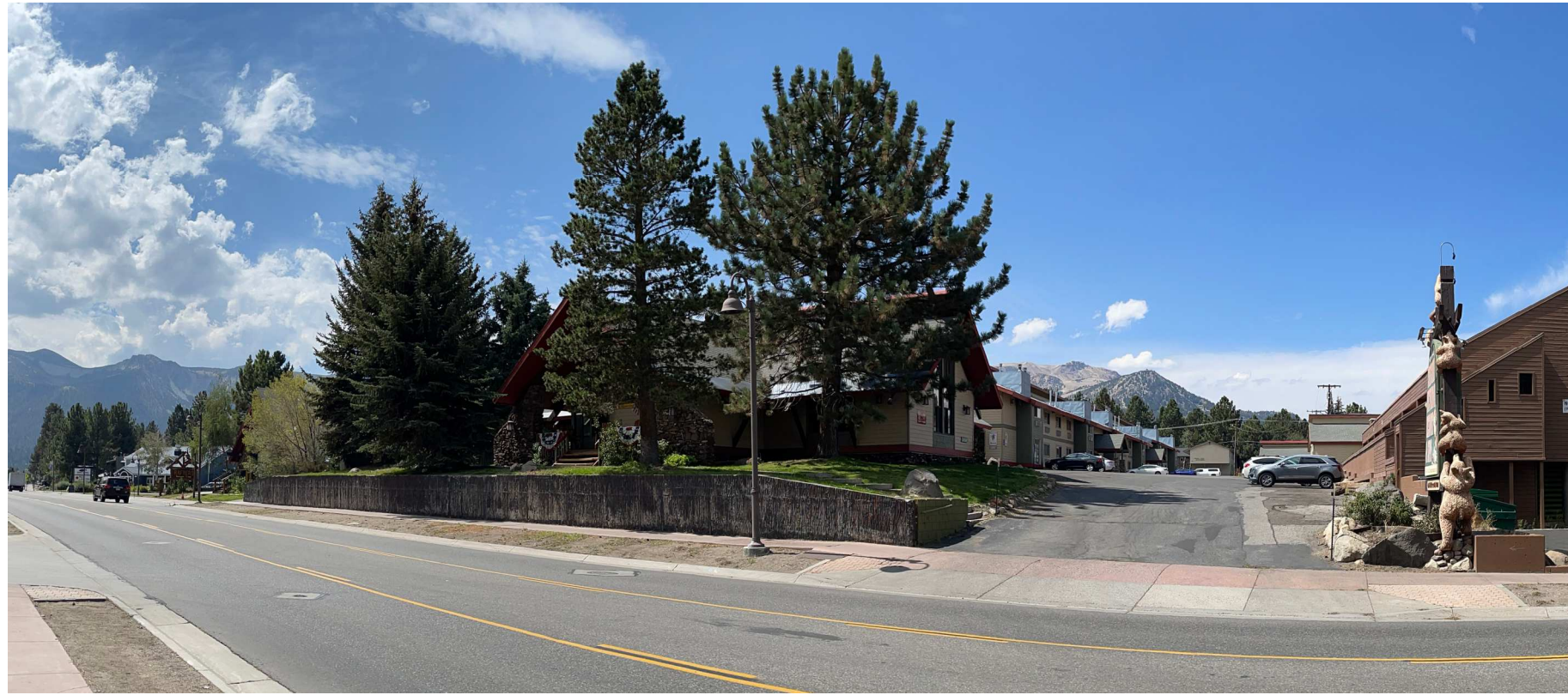
EXISTING CONDITIONS - OLD MAMMOTH ROAD
